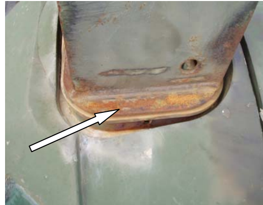
Ground edge of site housing on Control: Aug 11
